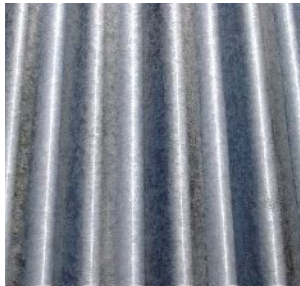
Corrugated Galvanized Steel Roof
